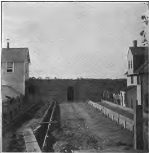
23.—Constructing house twenty-four feet wide; second step, making beds and walks.
